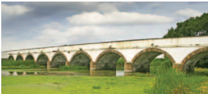
The Nine-holed Bridge
